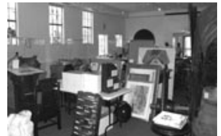
The mission side of the museum was completely dismantled for the renovation.
