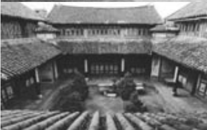
The Chinese have always built walls around their property. (Top) The outside view of a city's protective wall. (Middle) Neighboring houses, the only front doors are those which look out onto the street. (Bottom) A picture of the inside of a house. The house and its rooms create a wall around the central garden.
