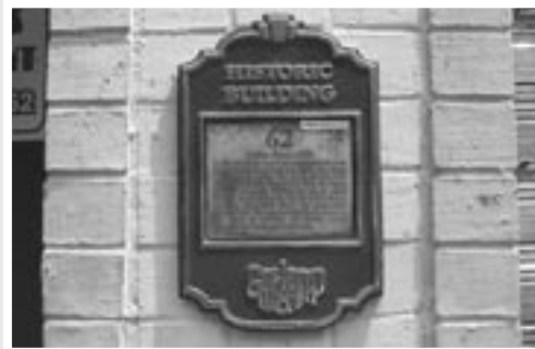
Deteriorating plaque on the Callan Hotel
